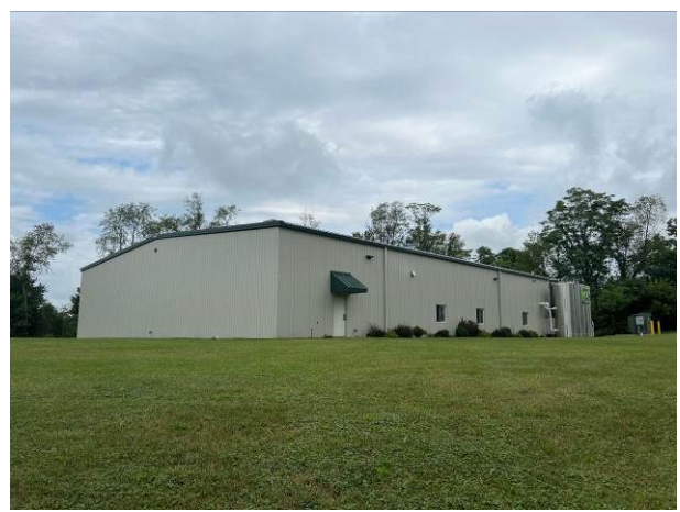
Front & South Sides of the Facility
