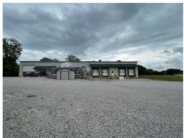
Rear of Facility – Loading Docks
