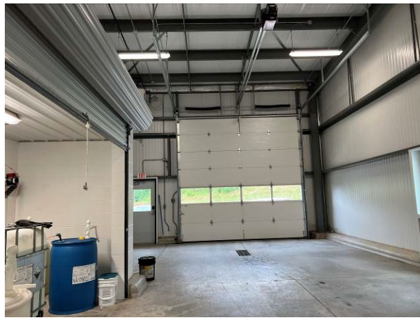
Drive through Receiving Bay
